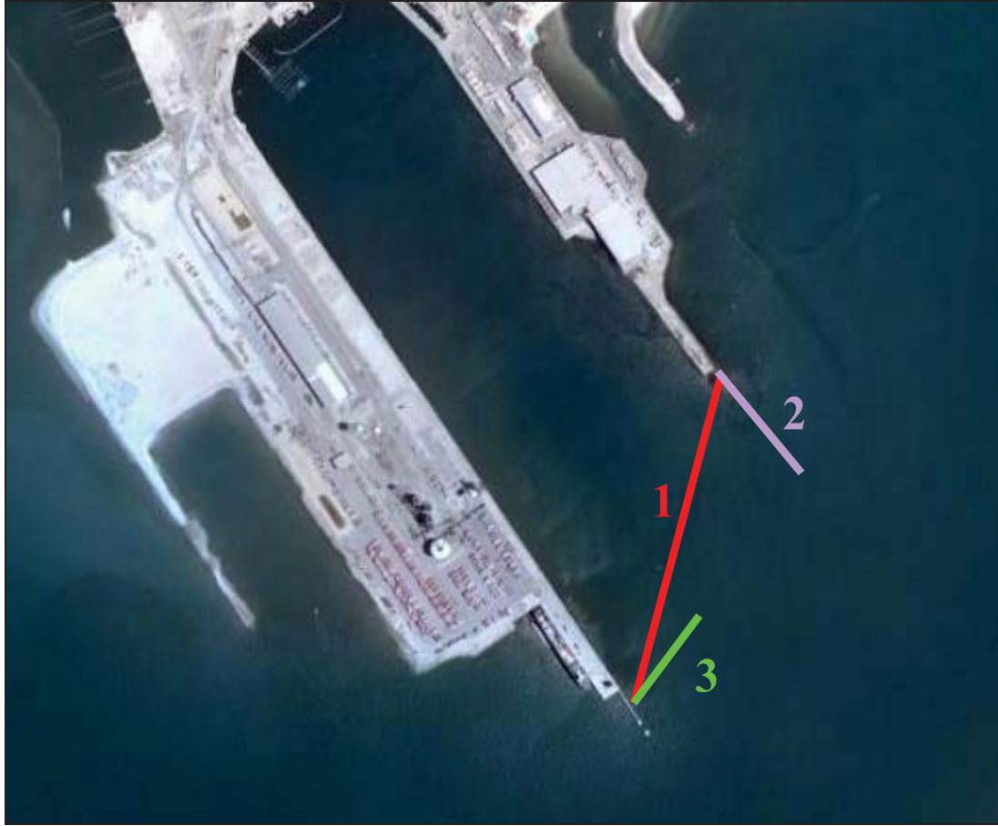
Figure 7-5 Locations for Possible Silt Curtains (Created with Google)
